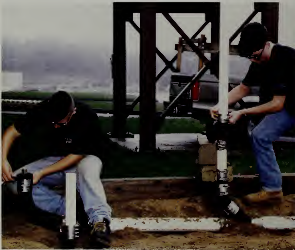
Kevin Porter and Justin Pierson work on a full bath rough-in outside the plumbing shop in "the underground pit."
